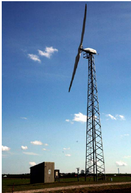
Figure 4: Gaia wind turbine
